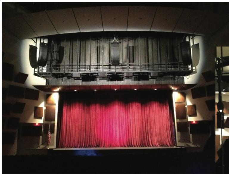
Left: The system includes 18 Bose RoomMatch loudspeakers installed in three arrays, plus eight RMS215 subwoofers.
